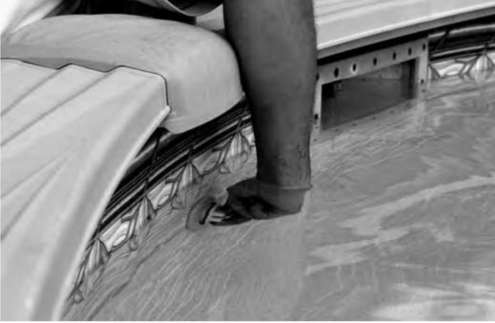
7. Take the hose end removed from pool return and connect to hose adaptor attached to the header. Tighten hose clamp with screwdriver.
