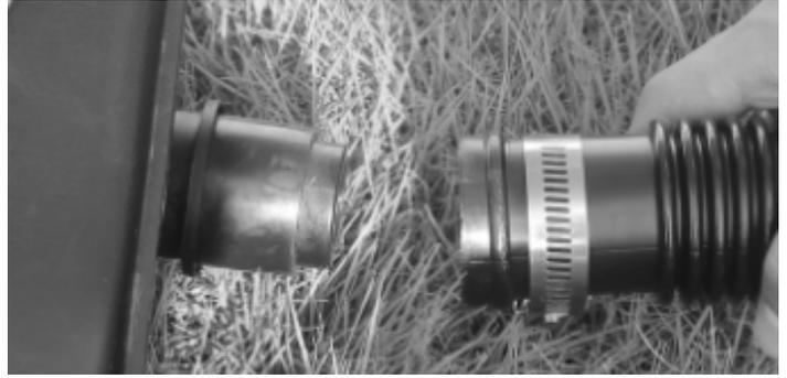
5. Make sure filter is turned off so no water flows out of the filter when disconnecting return hose from the swimming pool return and connecting to the solar heater.
