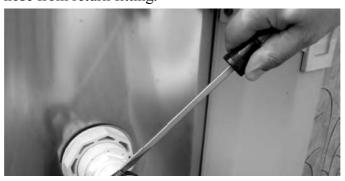
7. Take the hose end removed from pool return and connect to hose adaptor attached to the header. Tighten hose clamp with screwdriver.
