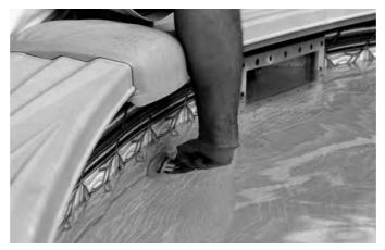
5. Make sure filter is turned off so no water flows out of the filter when disconnecting return hose from the swimming pool return and connecting to the solar heater.
