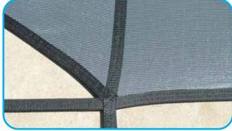
■ All covers are constructed with heavy duty polypropylene webbing and UV treated polyester thread. Strong enough to support the accidental intrusion of a stray animal or even a small car.
